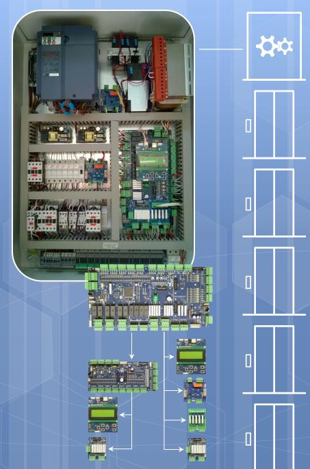
One of the main part of the elevator is its electronics. It is essential for both efficiency and durability, that are the basic principles of the new system «MYTA», which together with incredible versatility makes this product one of the top in the international market.
